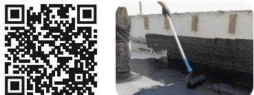
**CONSUMPTION** Minimum total consumption: 1.5 kg/m<sup>2</sup> (double layer)
