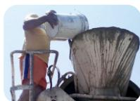
**CONSUMPTION** It is used at a rate of 2% of the cement ratio.
