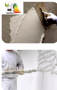
**CONSUMPTION** 13 kg: 3-3.5 m<sup>2</sup> for 1 cm thickness
