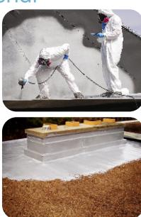
**CONSUMPTION** 1.00 kg/m<sup>2</sup> for 1 mm thickness
