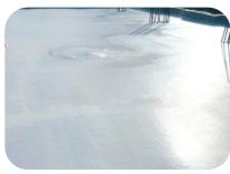
**CONSUMPTION** First layer: 0.75-0.9 kg/m<sup>2</sup> - Second layer: 0.75-0.9 kg/m<sup>2</sup>
