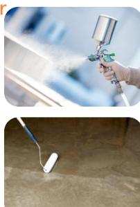
**CONSUMPTION** Depending on the porosity of the lower layer, it is applied with a brush or roller with a consumption of 100-200gr/m<sup>2</sup>.
