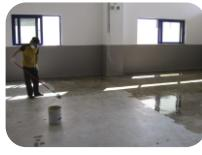
**CONSUMPTION** Depending on the porosity of the surface 350-500 gr/m<sup>2</sup>
